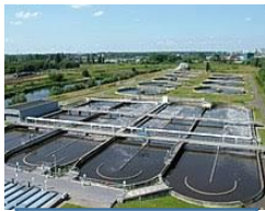
Waste water management
